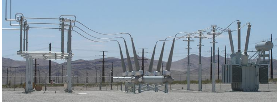
Harry Allen 500 kV Substation shunt reactor addition
